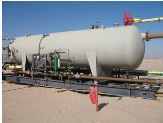
Figure 7: Typical Free Water Knock Out (FWKO)
