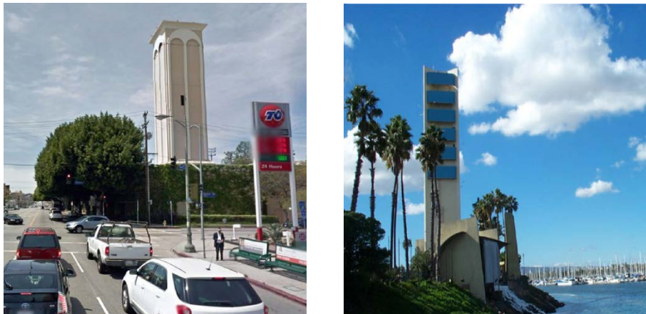
Figure 3: Typical Examples of Drilling Rig Coverings
